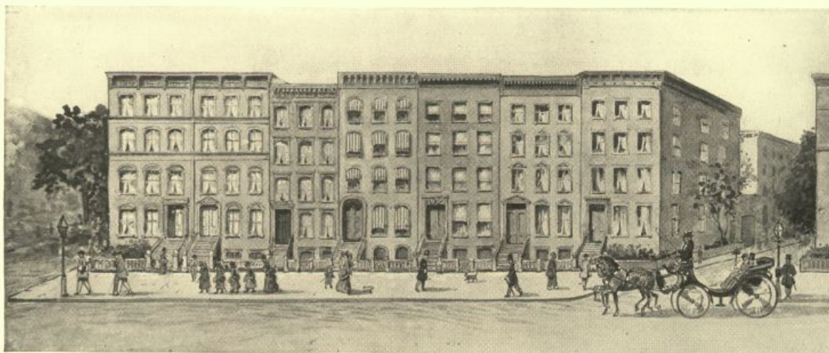
Fifth Avenue between 38th and 39th Streets, west side, about 1880
